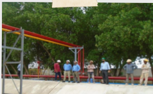
Ethanol Storage Tank
