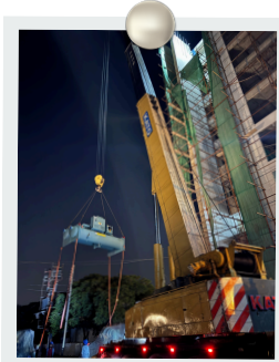
HBL Tower-2 Delivery
