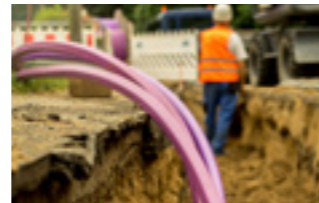
12 to 14 bar: Cable blowing and drilling
