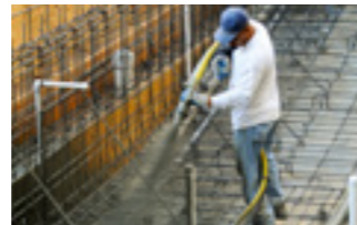
7 to 12 bar: Shotcrete applications
