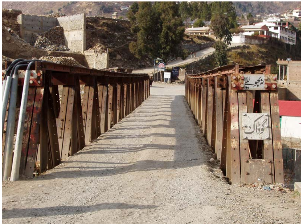
Photo 2: Temporary Bailey Bridge at Northern Outskirt of Madian Town (3.5 m wide)
